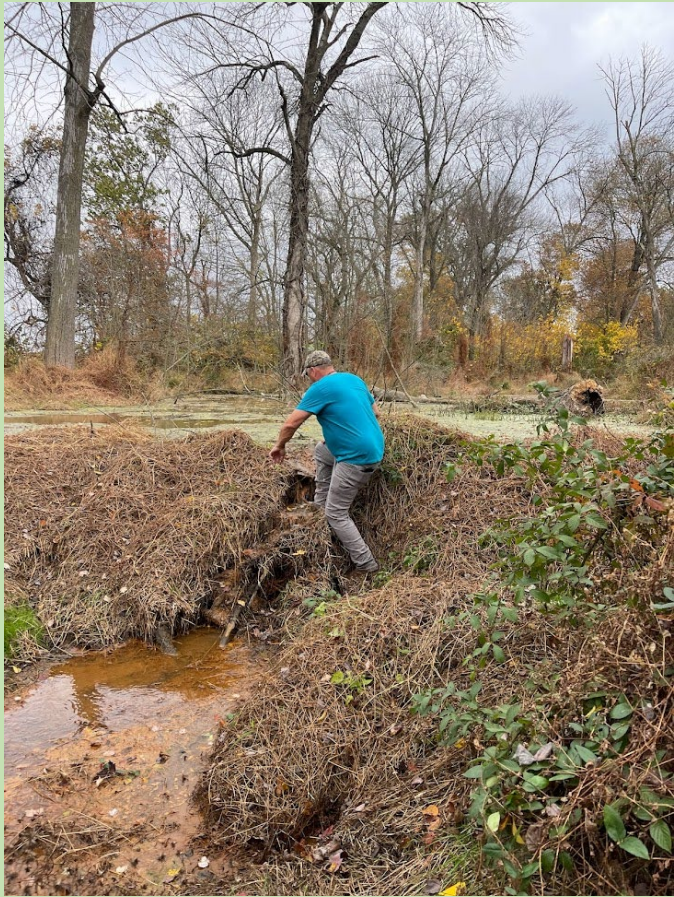
Point of failure forming on abandoned beaver dam
