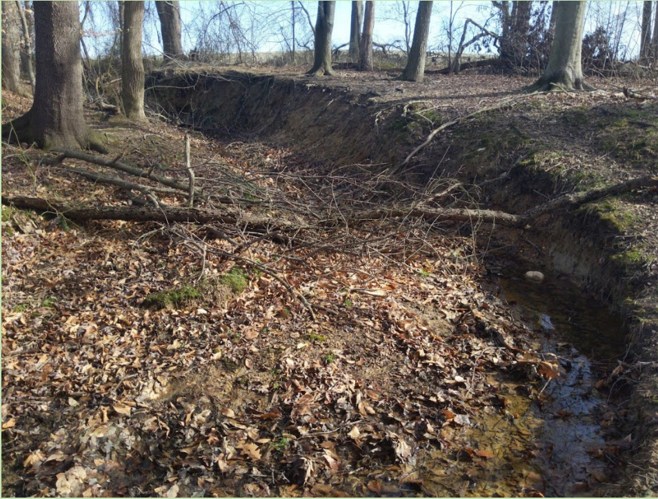
Headcut migrating toward field edge
