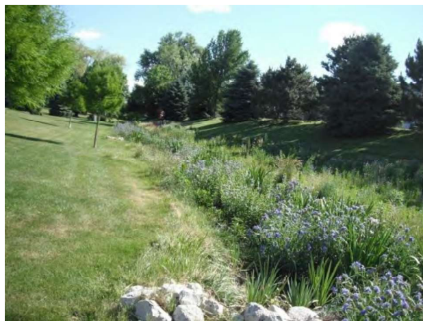
Figure 9. Example of vegetated open swale in Maryland.
