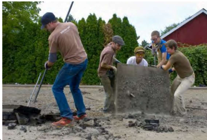
Figure 3. Depave, a non-profit from Seattle, WA, organizes volunteer groups to manually remove impervious surfaces.
