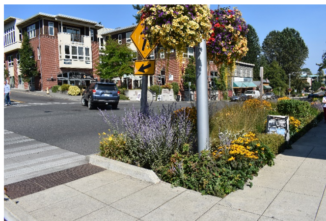
Green Street in Bainbridge, WA that has bioretentions installed into the sidewalk with curb cuts.
